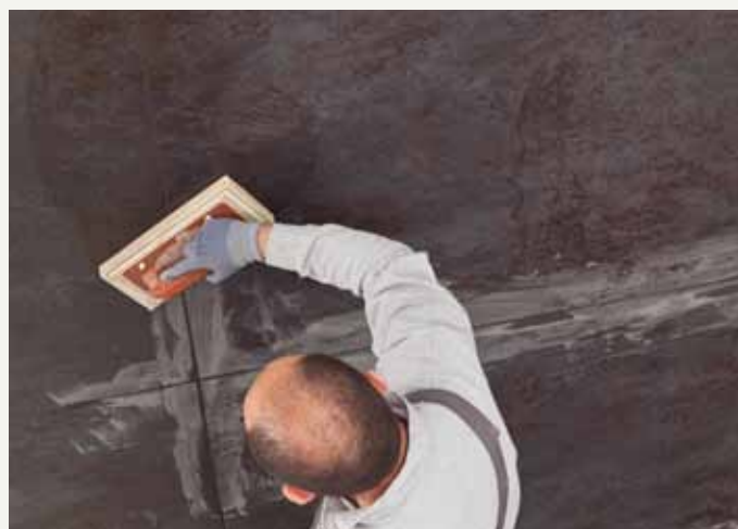
fig.39 / Stuccatura. / Grouting.
